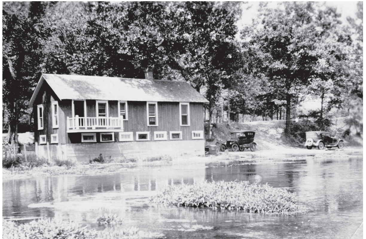
That is the original trout hatchery building, built in 1923 and then sold to the state in 1925. Until just the last few years, all the eggs taken were hatched and the trout fry (babies) were raised in the basement of this building. It is currently undergoing serious renovation at age 101.
