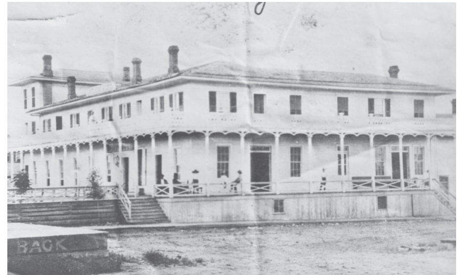
The fashionable Attaway Hotel in the 1880s was located next to the railroad before the Laclede Hotel taken on North Jefferson Ave.
